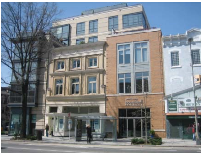
Figure 11: In this successful example, structures to the left, right, and above the center structure are additions.
