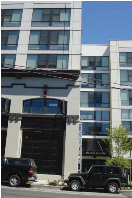
Figure 13: While the new structure is built above an existing character structure, the portion of the new structure that extends to the street helps to anchor the project to the streetscape.
