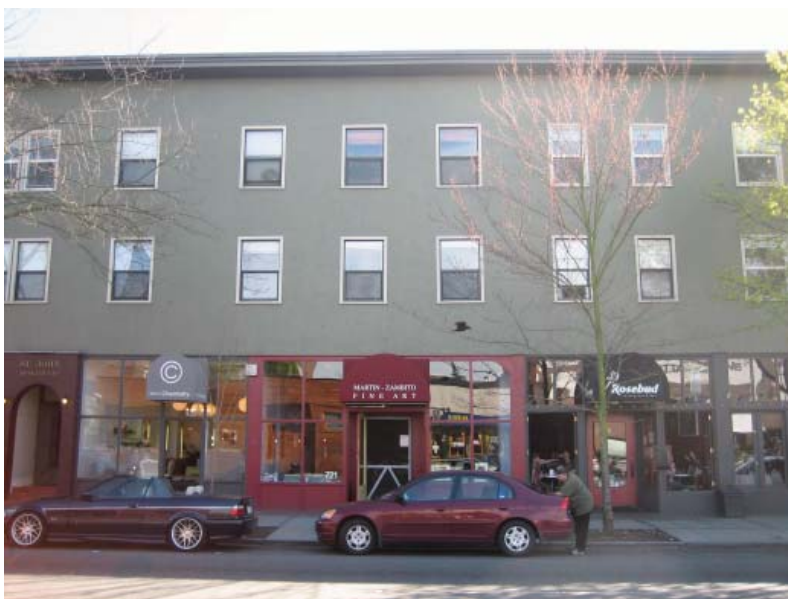
Figure 25: Transparent windows, retail modules and consistent entrances lend to human-scaled streetscape.
