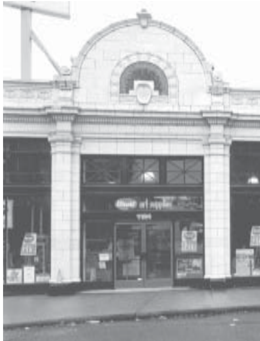
Figure 18: Context—pilasters, arched terra cotta cladding, parapet
